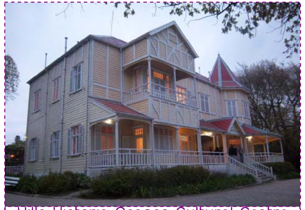
Villa Victoria Ocampo Cultural Centre
