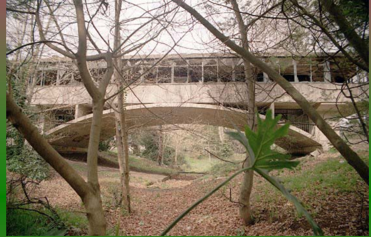
Side of the house
